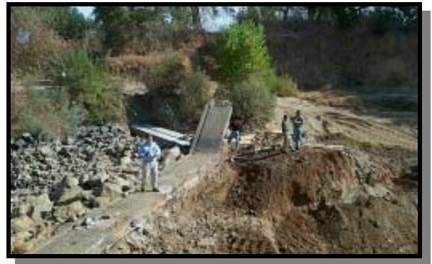
Blodgett Dam undergoing repairs.
