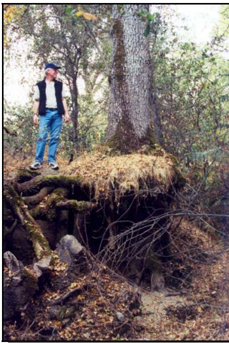
Ken Rood with Northwest Hydraulics Consultants, Inc. on top of unstable bank in Moco Canyon (photographer: Jeff Peters, Jones & Stokes).
